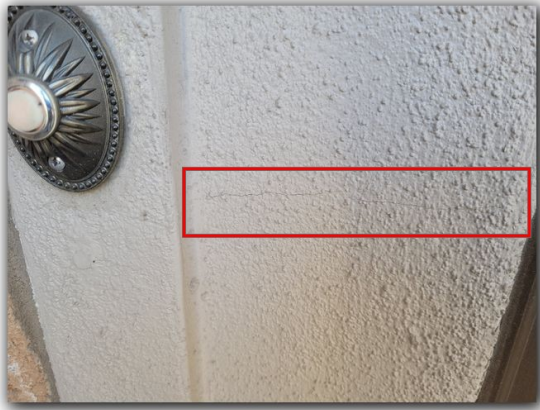
1- 2.4 Cracks - right side of stairs
