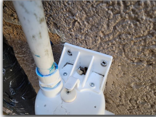
4- 1.4 Seal vent damper
