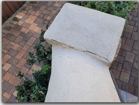
1- 2.4 Cracks - right side of stairs
